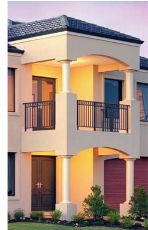
Galaxy (No. 138) with federation handrail.
