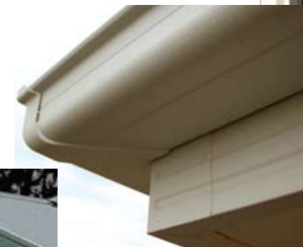
Quad Gutter and Fascia.
